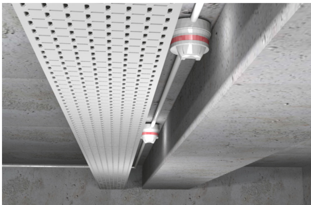
The sensor is obstructed by the lateral obstacles
